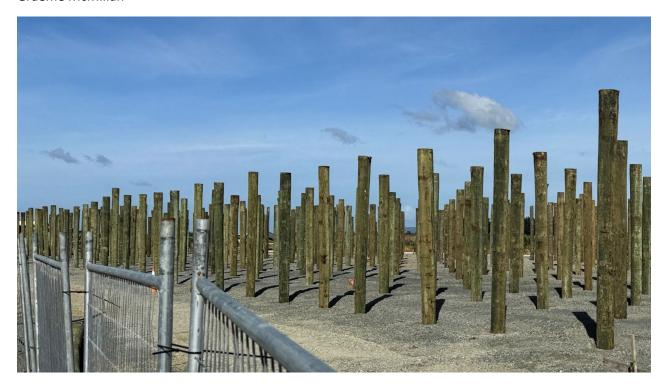
This is a lessons learnt project where timber moisture content created a strange modern art piece to be left on site to dry out due to the construction issues it caused.
